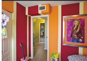
THE SECOND-FLOOR BEDROOM shows soffit above the door, which hides the air conditioning duct. Note the register that throws conditioned air across the ceiling.
